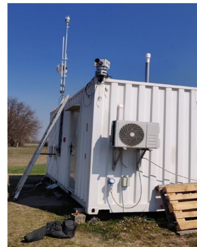
Skyspec-2D system at San Pietro Capofiume
